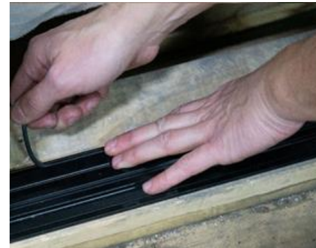
7. Interlock tracks with sill . Insert spline into groove.
