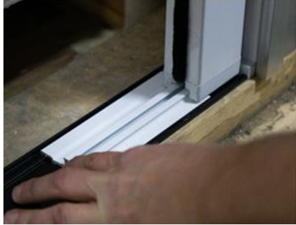
1. Remove track cut-off.
