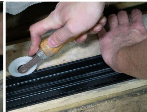
7. Interlock tracks with sill . Insert spline into groove.
