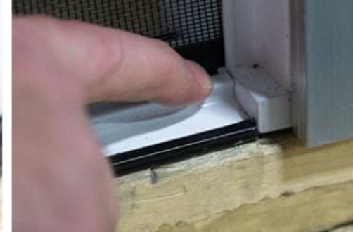
4. Push fully against housing – no gaps .
