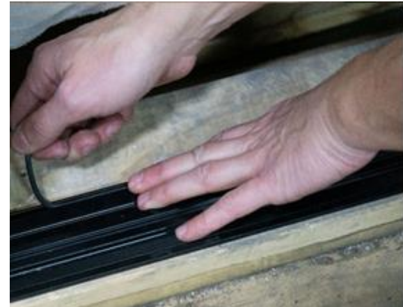
7. Insert spline into groove.
