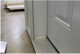
Moulding extends past the threshold
